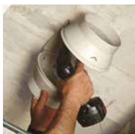
Fix the support bracket.
