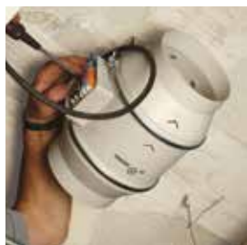
Carry out the wiring connections.
