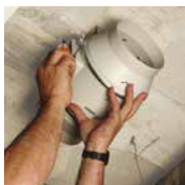
Place the impeller and motor.
