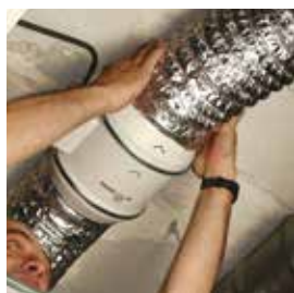
Connect the ducts.
